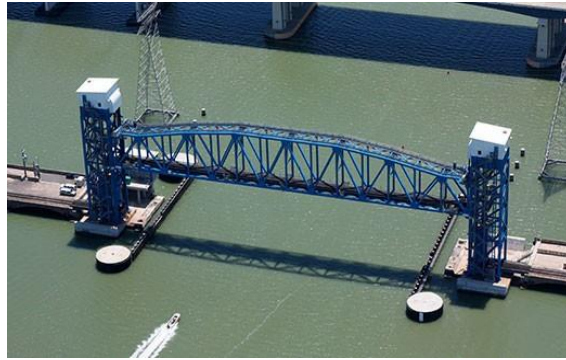
Galveston Causeway Railroad Bridge
